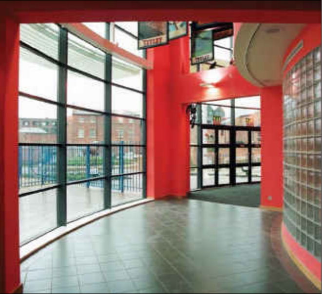
Ground Floor Framing with Entrance Doors
